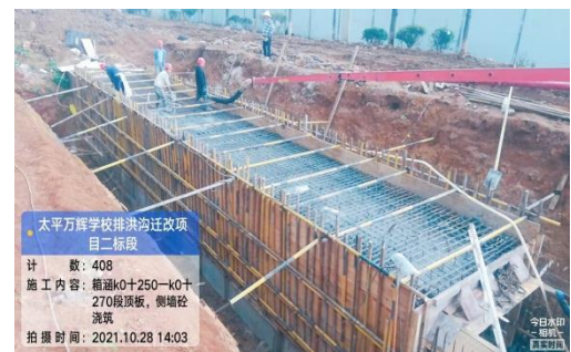
墙身及顶板浇
